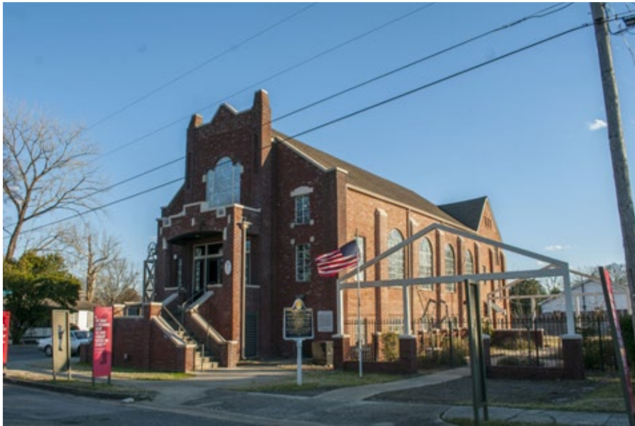
Figure 37: Bethel Baptist Church fully restored | Source: Birmingham Civil Rights Institute.
