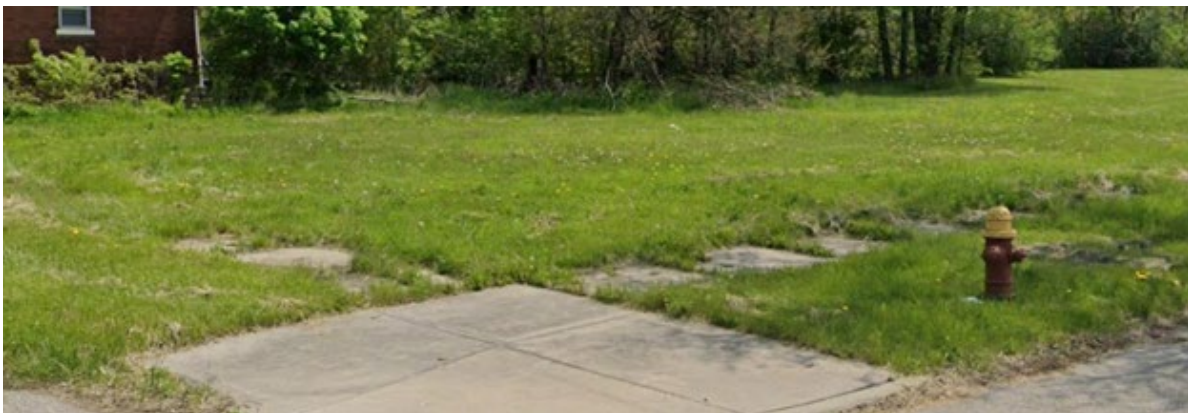
Figure 35: Sidewalk at Antoinette St. & Wabash St. | Source: Google.
